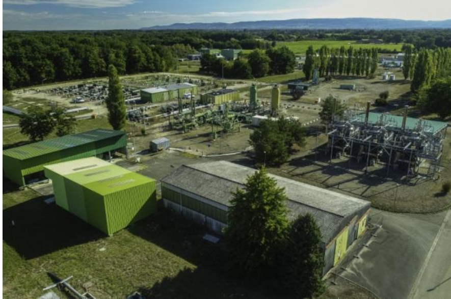
Fig.20 : HyPSTER – Hydrogen underground storage in salt caverns
