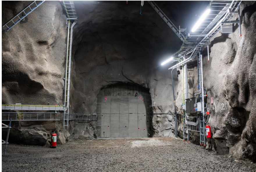
Fig.21 : HyBRIT – Rock caverns storage – Underground, fossil free hydrogen gas storage facility – Svartöberget Sweden
