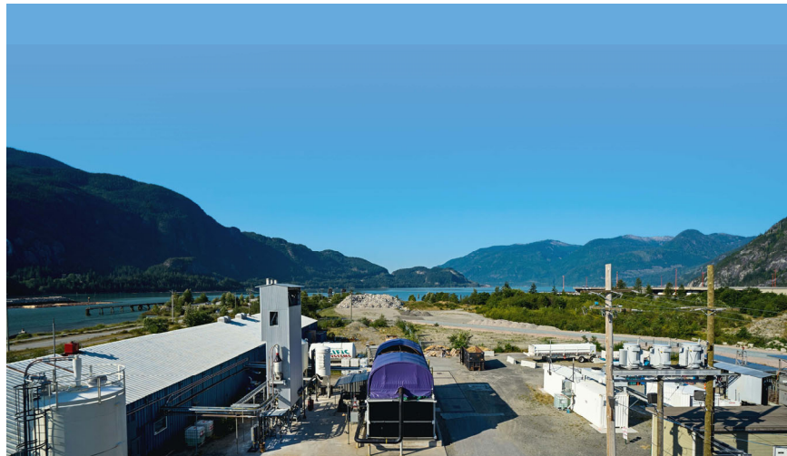
DAC Pilot Plant in Squamish, Canada. Source CE
