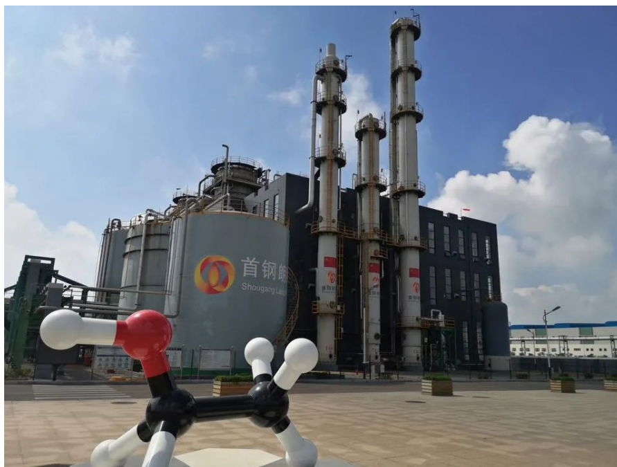
Lanza Tech Ethanol Plant Beijing Shougang, China
